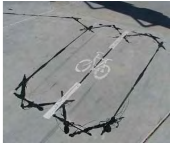
Bicycle loop detector stencil
